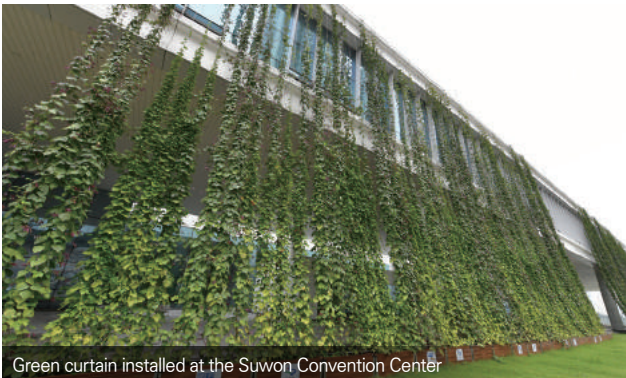
Green curtain installed at the Suwon Convention Center
